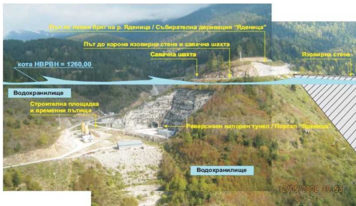
Fig. 7. "Yadenitsa" construction site
