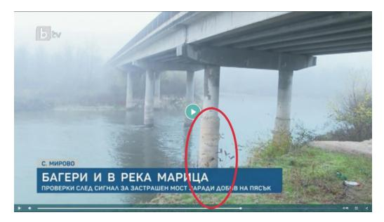
In the ellipse on the photo the original cast in situ pile is visible. The pointer shows the upper end of the pile at the time when it was casted. This was the original level of the bottom of the riverbed back then.
