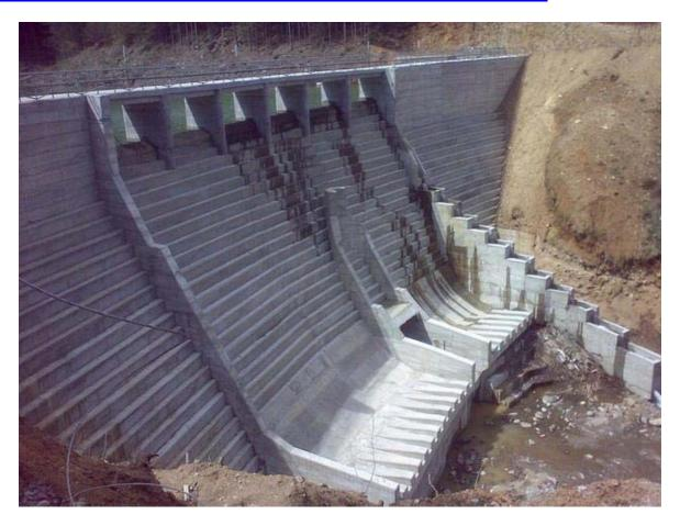
This picture displays the most stupid fish pass on Earth. Should any fish manage to pass through - it will immediately be killed by the abrupt change of about 10 meter difference in water pressure. Thankfully no fish would be so stupid, as incompetent are the fish pass designer and MOEW personnel that has assessed this facility acceptable for operation. Sadly, this is the fourth HPP barrage slicing
