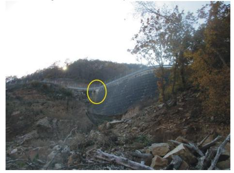
This picture, taken from the riverbank, shows the north sump. Big exhaust pipes (indicated in the yellow ellipse) are clearly visible at the left hand top corner of each barrage, with one possible purpose: to serve as spillways. The entire mining area, including the sumps, can be viewed in this video, shot with a drone: https://www.youtube.com/watch?v=pEvCHLi846c The south sump below the *Ada Tepe* Waste Management Facility is more clearly visible in this video at 4:20:
