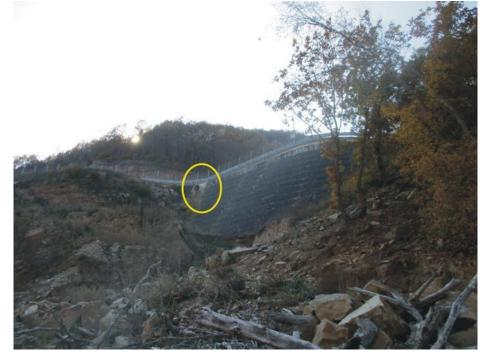
This picture, taken bottom up from the riverside, shows the north sump. Big exhaust pipes /in the ellipse/ are clearly visible at the left hand top corner of each barrage, with one possible purpose: to play the role of spillways. The entire mining area, including the sumps, can be watched in the following video, shot with a drone: https://www.youtube.com/watch?v=pEvCHLi846c
